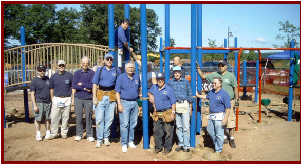
Among the volunteers working over the June 23-24 weekend to ready the playscape at the new Nayaug Elementary School in South Glastonbury for opening day of school were brothers of Columbia Lodge No. 25 A.F. & A.M. Shown from the left are Pete Gambardella, Rob Brautigam, Ward Edgerton, Walt Grube, Rich Beebe (above on the bridge), Skip House, Bob Flint, Geny Thompson, Don Wills and Mike Vose with several other citizen volunteers, in the back ground, working on Saturday morning.
